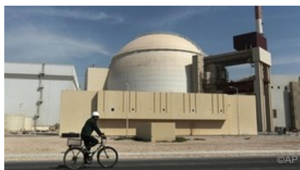
Bushehr nuclear power plant, Iran
